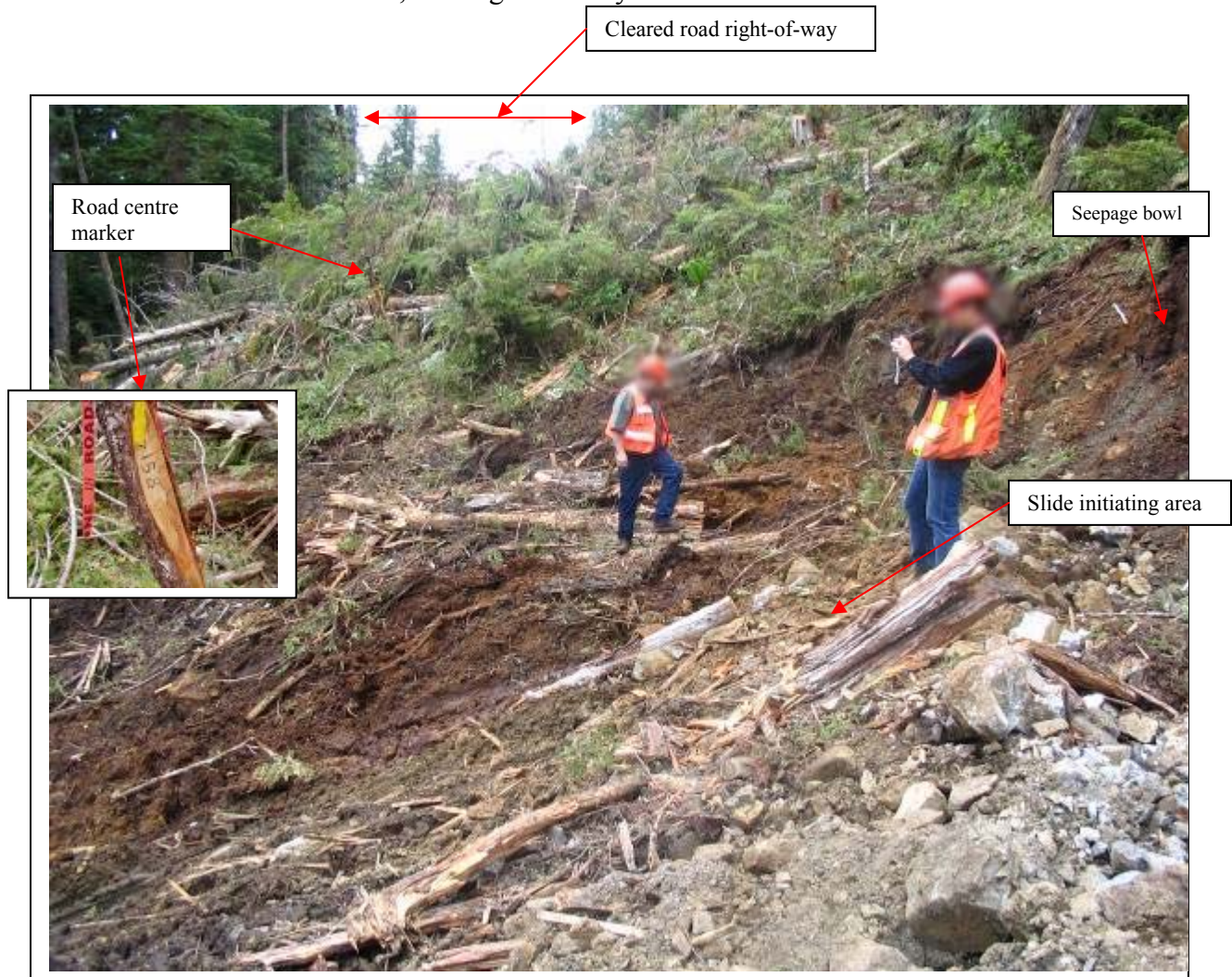
Photo 1: This photo taken after the incident shows the location of road centre marker.
