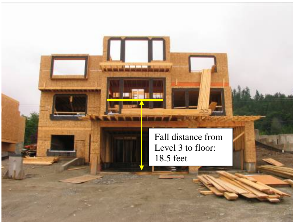
Figure 3: Distance from Level 3 to concrete floor.
