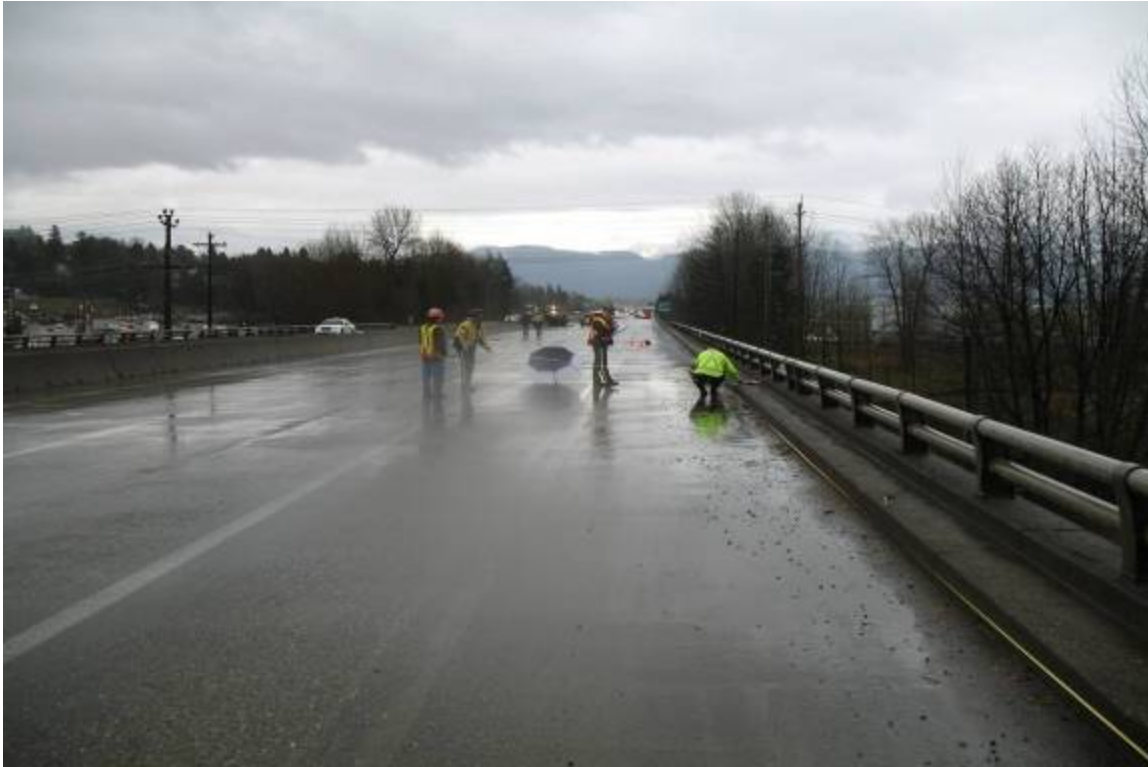
Figure 8: The concrete overpass, showing the road shoulder.
