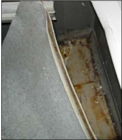
Asbestos-containing flooring
