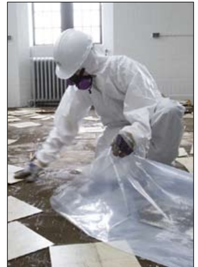
Worker removing asbestos floor tile
