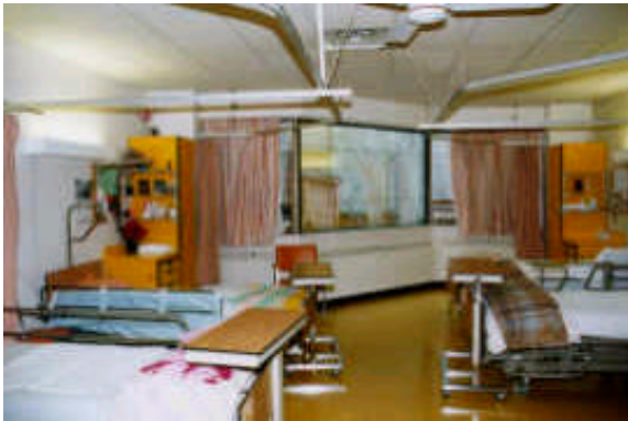
Typical 4 bed room after ceiling lift installation
